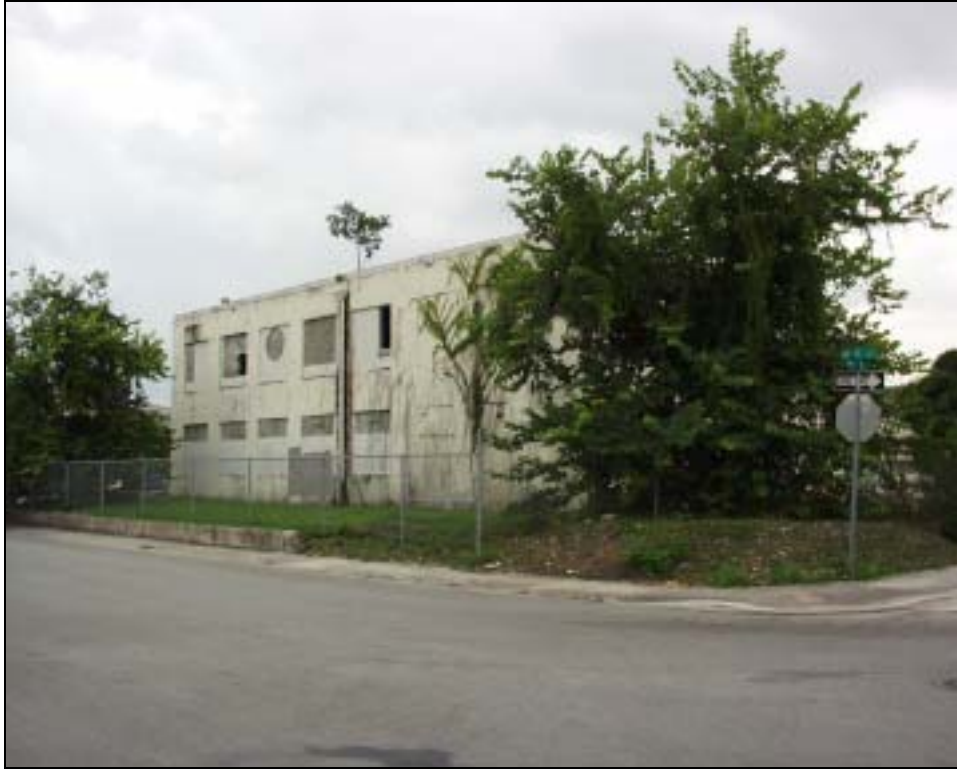
Figure 3: North Elevation, Facing Southeast Photograph taken by Amy Strelman, August 2002
