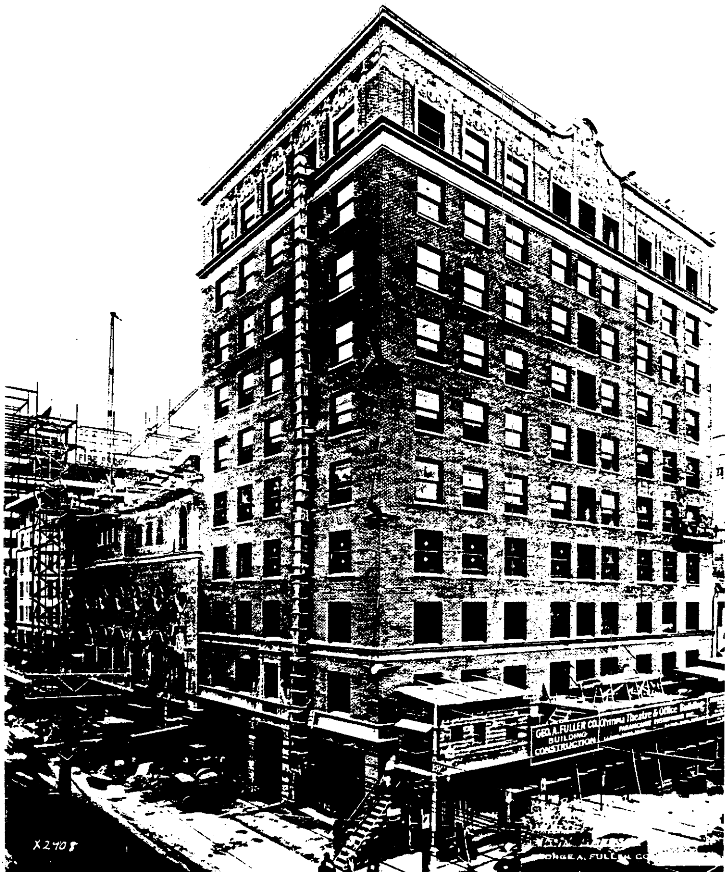
Olympia Theater and Office Building 174 E. Flagler Street East and north (front) facades (building under construction) 1925 (Courtesy of City of Miami Off-Street Parking Authority)
