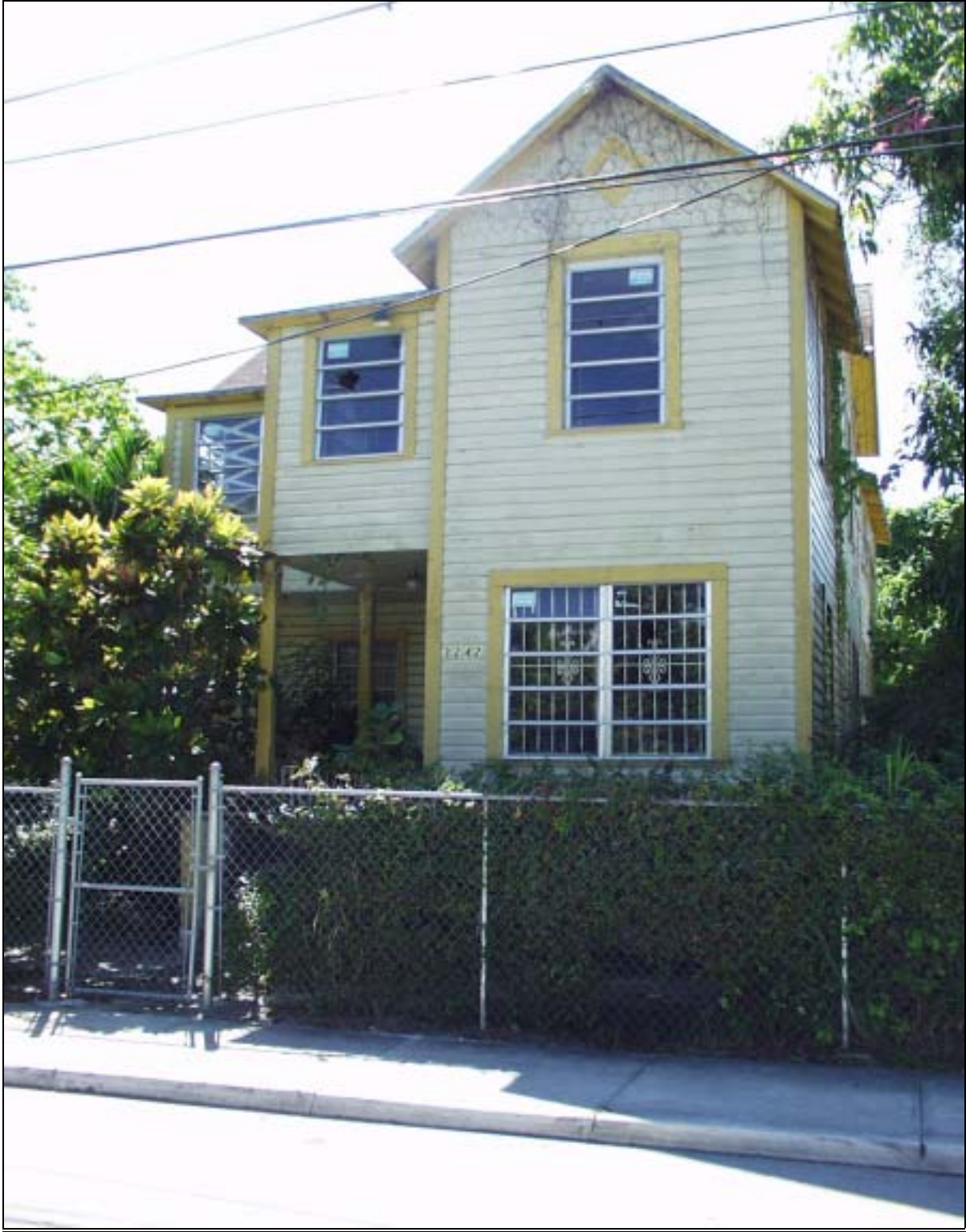
E.W.F. Stirrup House 3242 Charles Avenue North and west façades 2002
