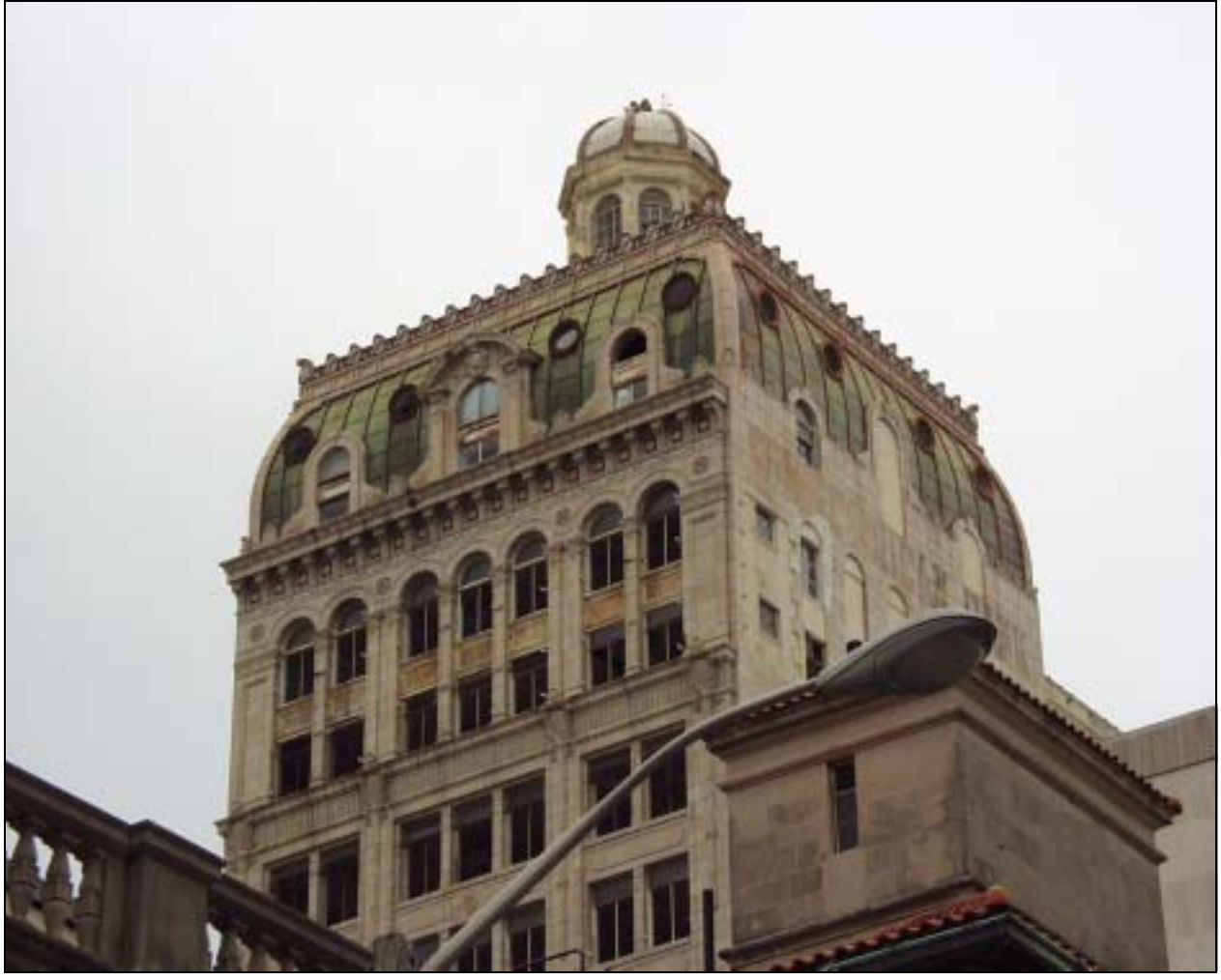
Security Building 117 NE 1 st Avenue South and west façades 2002
