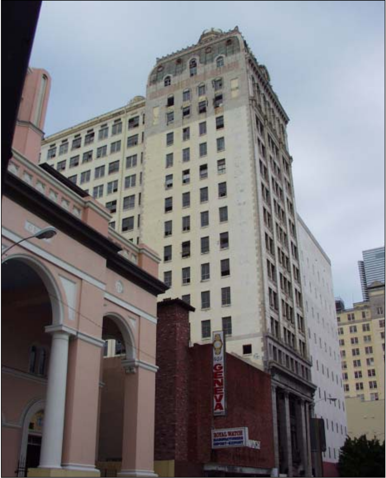
Security Building 117 NE 1 st Avenue North and west (front) façades 2002
